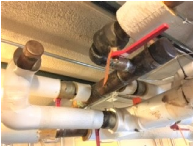
Plumbing layout for three boilers
