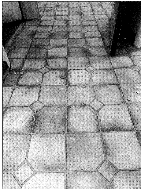
View of Square Pattern Linoleum and Yellow Mastic over White Floor Tile and Yellow Mastic (HA3)
